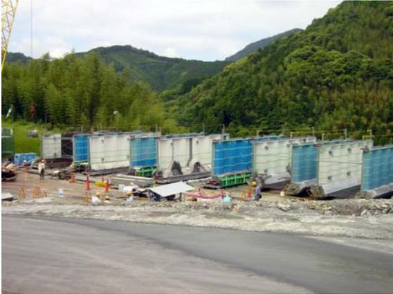
**Photo. 3.** Precast members for the corrugated steel and concrete lower flange
