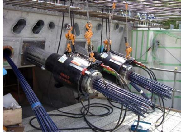
**Photo. 4.** The anchorages for the cables provided with shim plates
