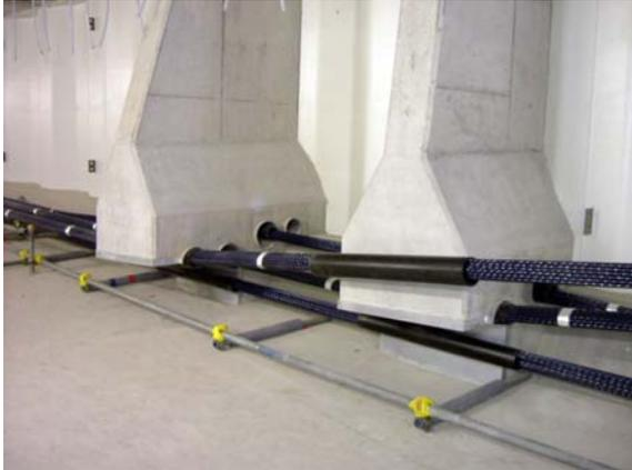
**Photo. 7.** The deviators for the reused cables
