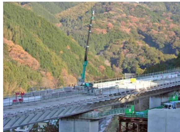
**Photo. 6.** The placement of PCPca-panels for the wing slab
