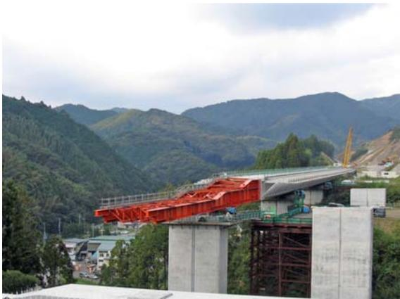
**Photo. 5.** Overall view of the incremental launching process
